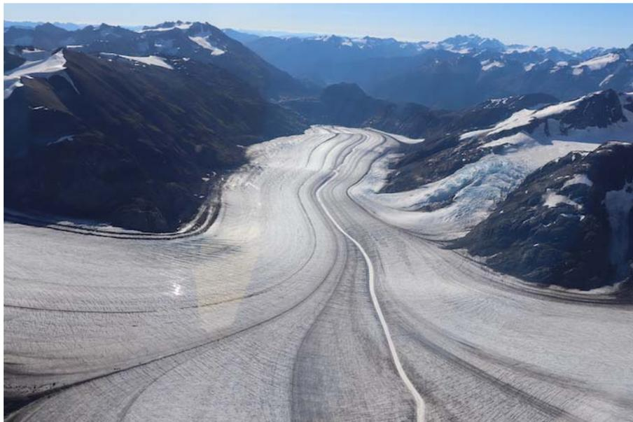
A supply road built overtop of a glacier, leading in and out of the Brucejack Mine
